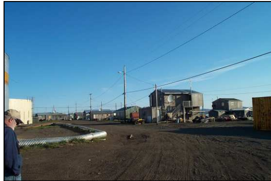
Typical structures in Kivalina
