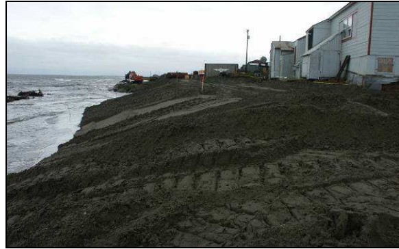
Corps Project Under Construction in 2005
