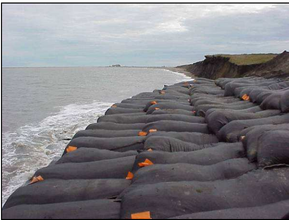
Corps Gravel Bag Revetment in 1999
